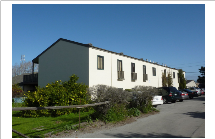
Image 4. South elevations, two-story office building at rear of property (ARG, January 2011).
