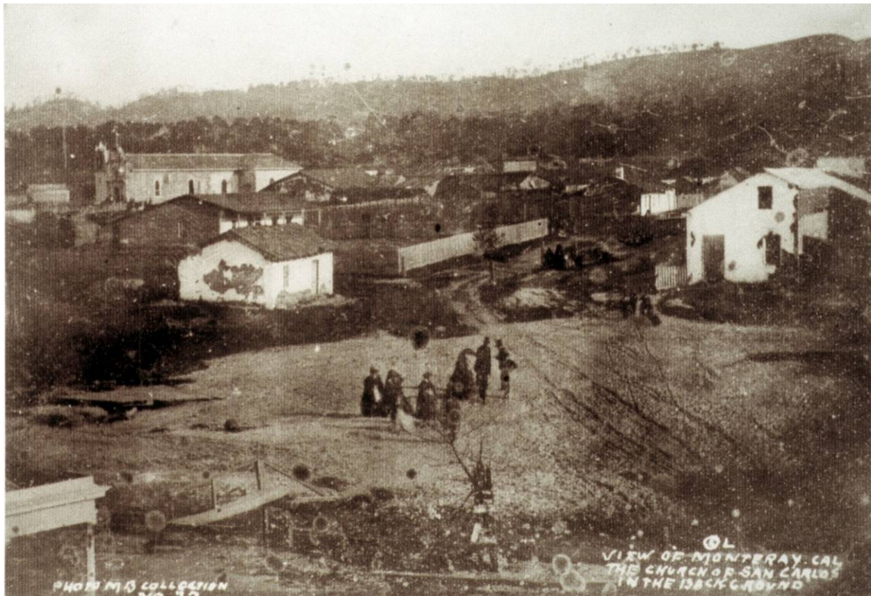
Figure 7-2. Early view of Abrego Street at Pearl Street, taken from upper story or roof of the Washington Hotel. Casa Abrego is visible on the right. The Royal Presidio Chapel is in the background, with 1859 transepts visible. Note the planks over Hartnell Gulch (courtesy Monterey Public Library, California History Room).
