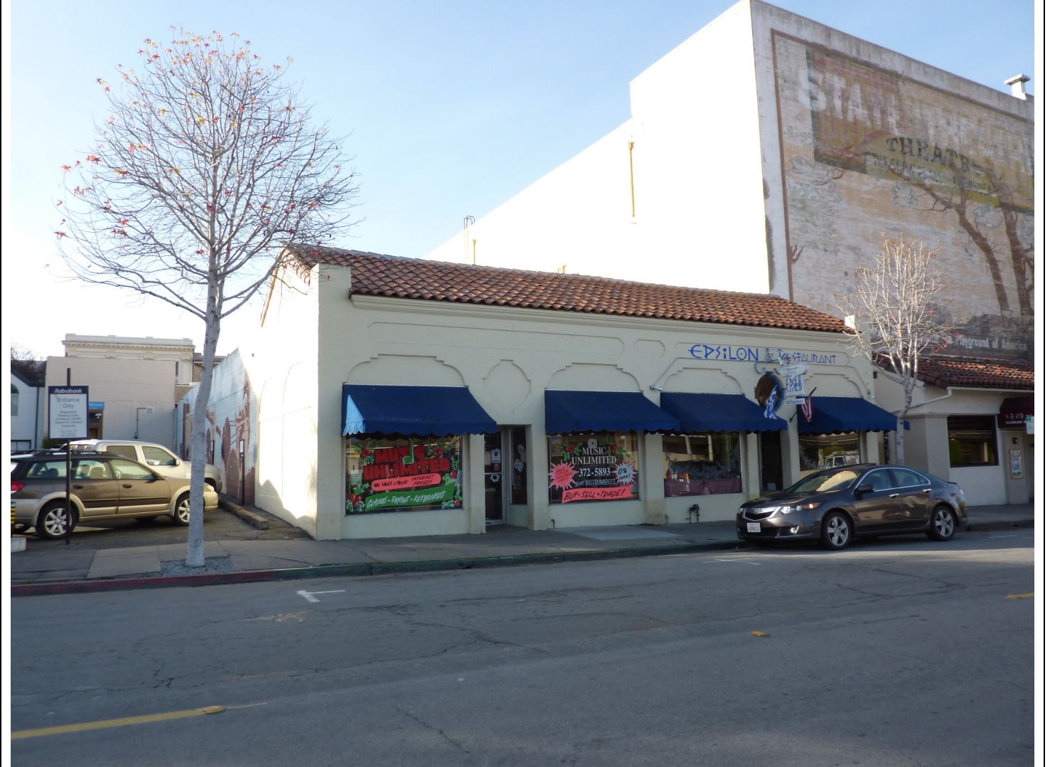
East (422 Tyler Street) elevation (ARG, January 2011).
