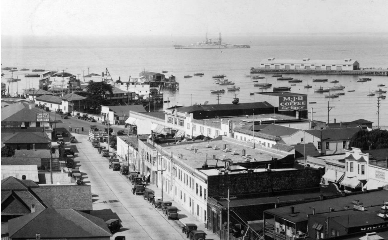
Figure 9-7. Portion of 1927 panorama showing lower downtown and the end of the New Wharf (A.C. Heidrick, photographer, courtesy Monterey Public Library, California History Room).
