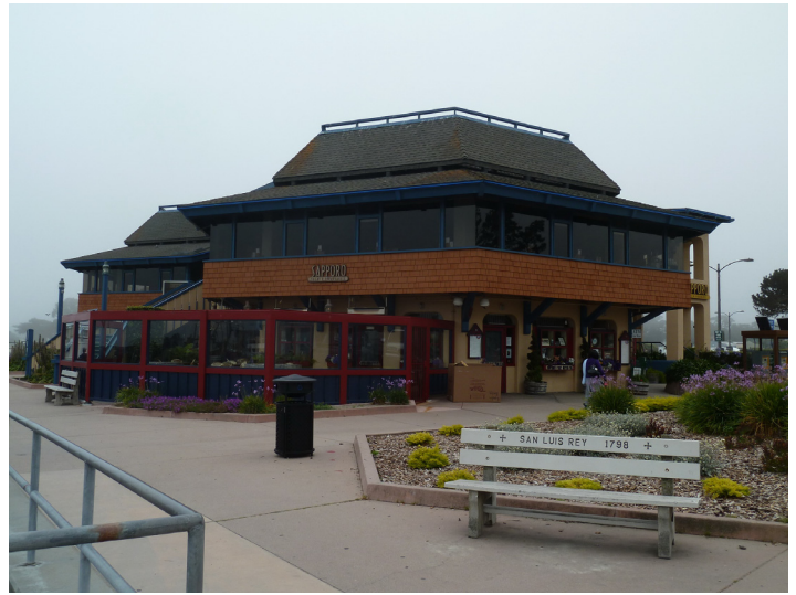
Image 7. North and west elevations, southern restaurant building (ARG, January 2011).
