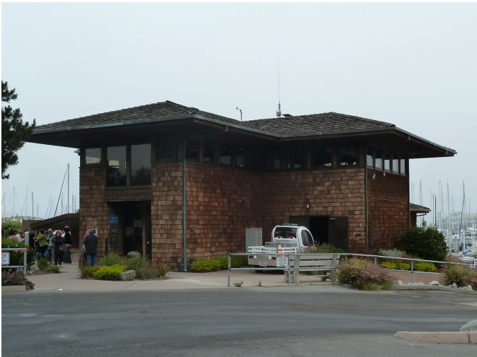
Image 8. South and east elevations, harbormaster building (ARG, January 2011).
