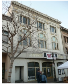
Regency Theater/BPOE Building (1917) 426 Alvarado Street
