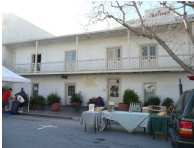
Osio-Rodriguez Adobe (1849) 380 Alvarado Street
