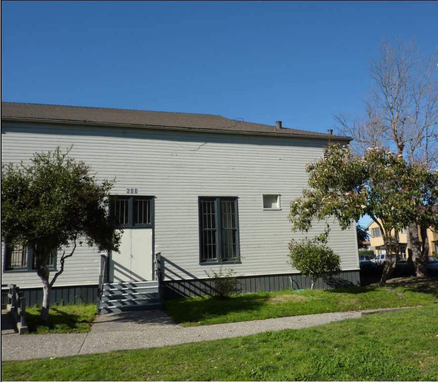
Image 3. Northern portion of east elevation of gymnasium (ARG, January 2011).
