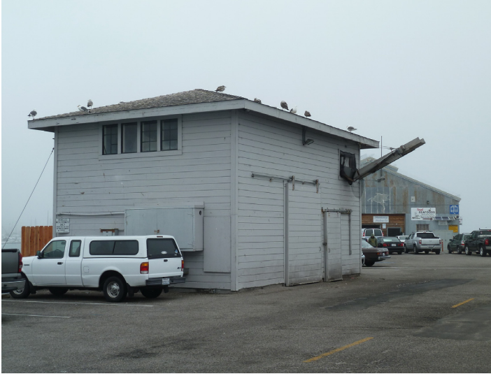
Image 2. South and east elevations, northern ancillary building (ARG, January 2011).
