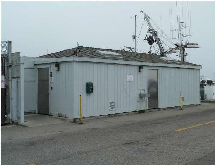
Image 4. South and east elevations, public restroom facility (ARG, January 2011).
