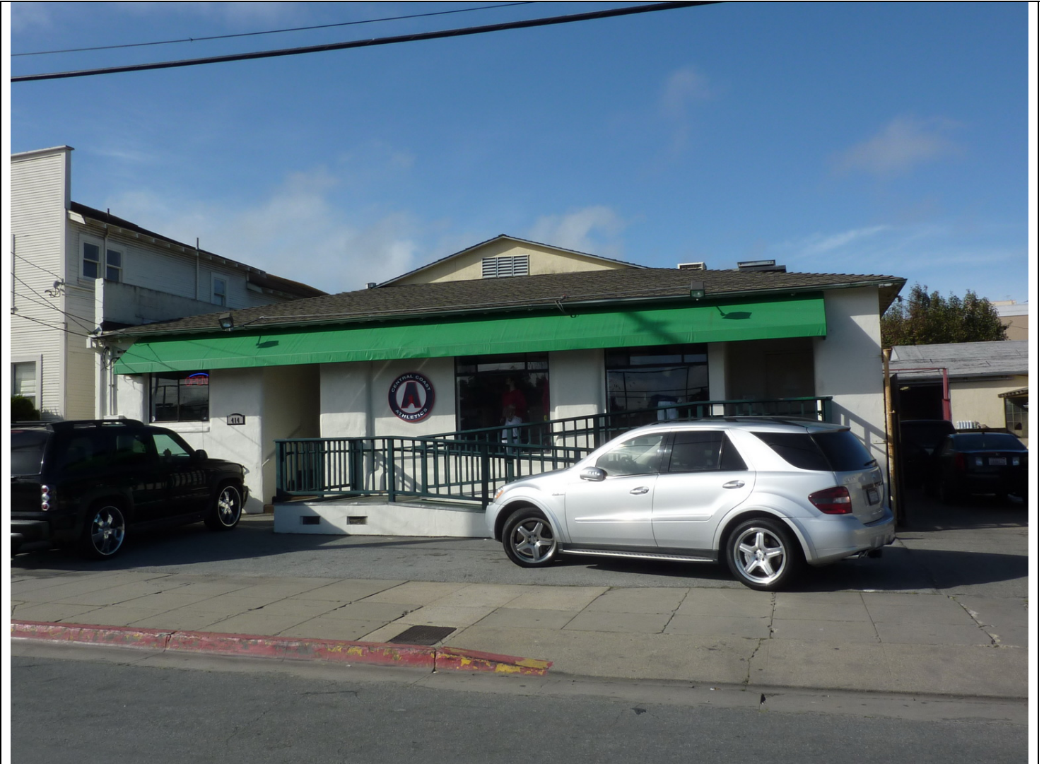
East elevation of building at 414 Adams Street (ARG, January 2011). This building appears to date from c. 1955. It has been extensively altered and retains insufficient integrity to be potentially historic (6Z).
