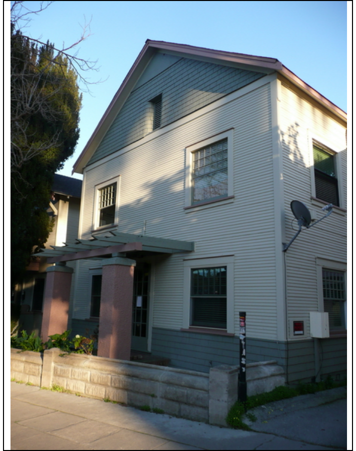
Image 3. North elevation, 579 Polk Street (ARG, January 2011).
