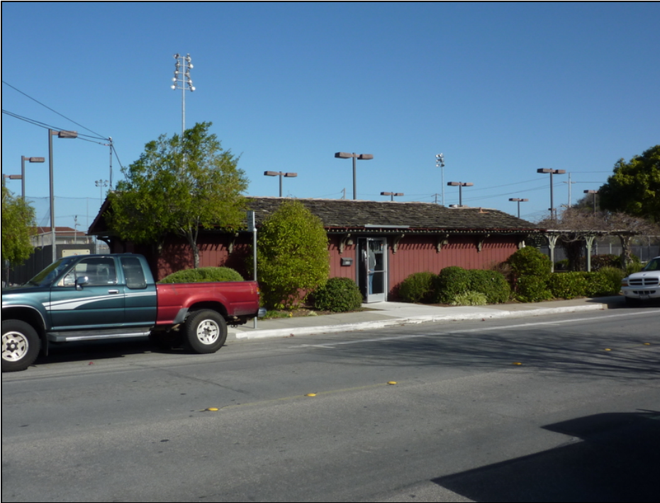
Building at south end of park, south elevation (ARG, January 2011).
