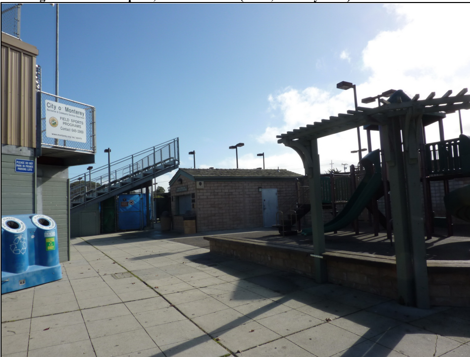
Bleachers, CMU building, and playground, looking east (ARG, January 2011).
