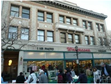
A.R. Underwood Building (1912) 416 Alvarado Street
