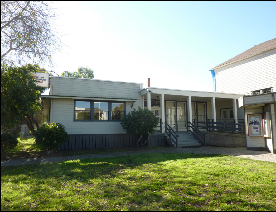
Image 2. Portion of north elevation (ARG, January 2011).
