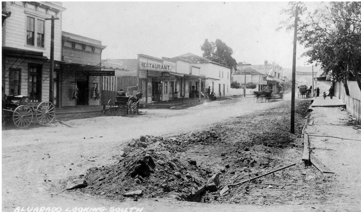
Figure 8-1. 1887 view of sewer line trench being dug along Alvarado Street (C.W.J. Johnson, photographer, courtesy Monterey Public Library, California History Room).
