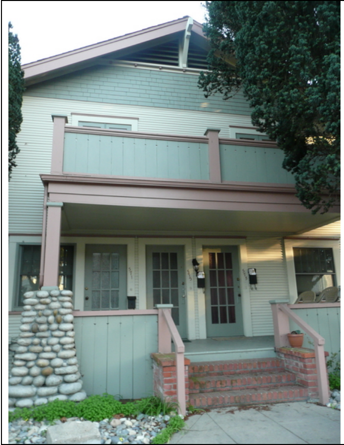
Image 2. North elevation, 571-575 Polk Street (ARG, January 2011).
