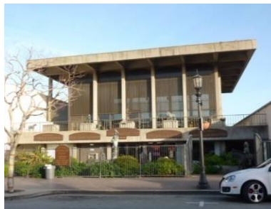
International Style: Monterey Savings and Loan (1962), 449 Alvarado Street
