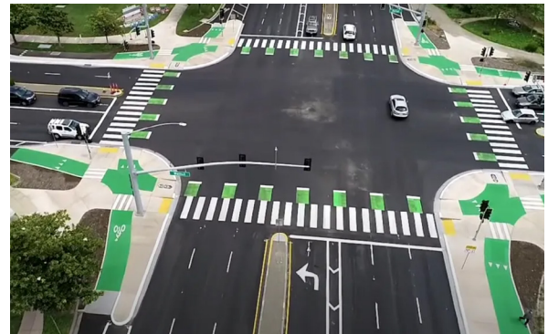
Protected Intersection in Fremont, CA - Source: StreetsBlog SF
