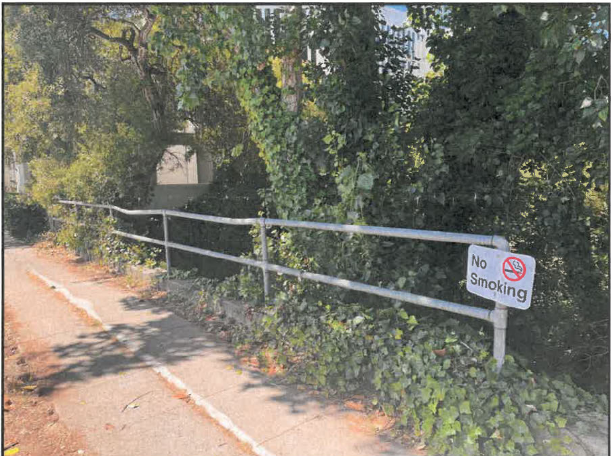
South Side of Hartnell Street - Upstream
