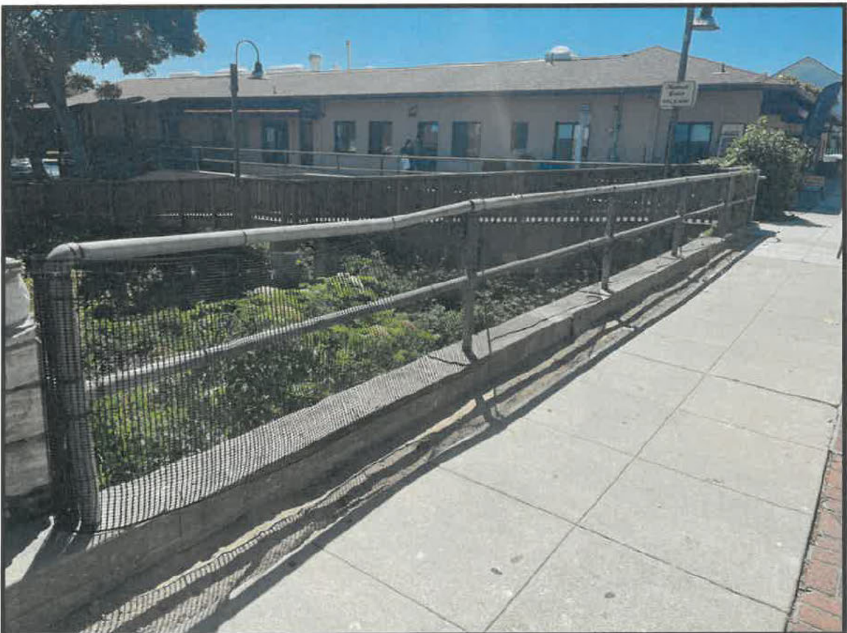
North Side of Hartnell Street – Downstream
