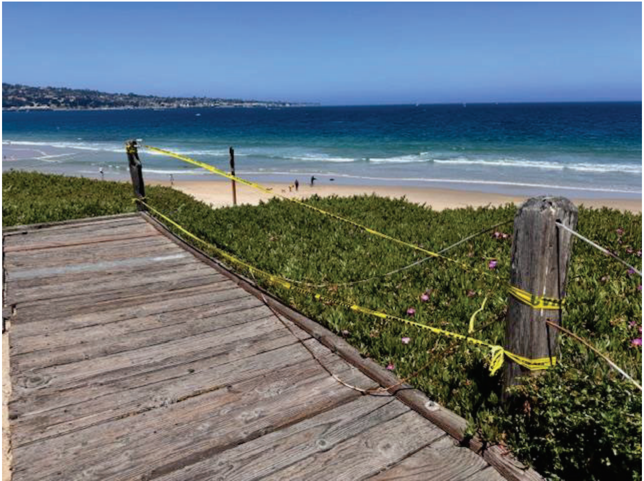
BEFORE – broken cables/rotted posts & AFTER – split rail fence protecting dunes habitat
