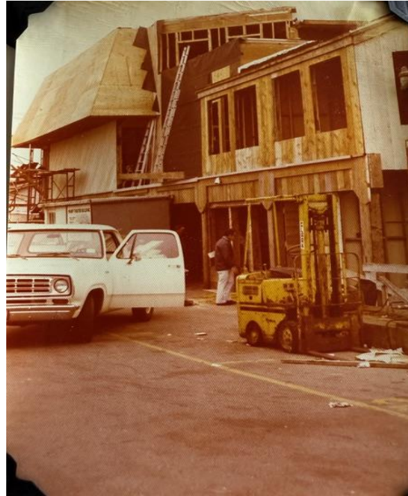
Construction of the Wharf Theater with Angelo DiGirolamo, builder. 1975.
