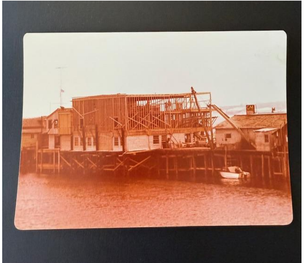
Construction of the Wharf Theater by Angelo DiGirolamo, builder, and Bruce Ariss, Designer/Builder. 1975.
